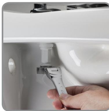
Tighten with Spanner
